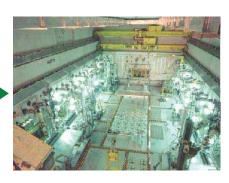
After removal from the VTR core (and possible temporary storage in the VTR facility), test assemblies would be transferred to a post-irradiation examination hot cell facility. The assembly would be cleaned and the test specimen removed. Initial post-irradiation examination would be performed in this facility.
